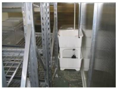
Figure 7. IAR wastewater collection tub with sump pump below.
